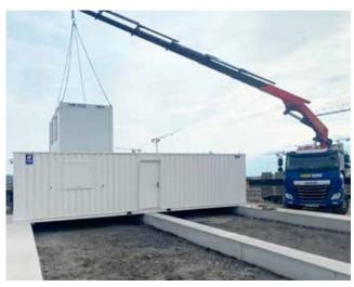
Link space units can be stacked side by side up to 3 storeys high with external staircases used to access the link corridor. These units offer the most cost-effective way to provide large accommodation space in a quick time frame so you can start work on site immediately. Linked units can be configured to suit your layout requirements including offices, canteens, drying rooms, meeting rooms along with toilets and showers.
