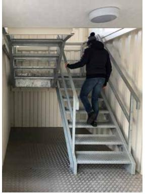
These purpose built staircase modules provide quick and easy access to stackable modular building configurations either 2 or 3 floors high. Internal and external stairway options are available and have been deigned and manufactured to allow quick erection on-site, ideal for a wide range of applications on small or large construction or industrial sites.
