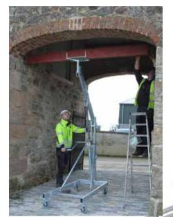
The unique beam lifter is an easy to operate lifter suitable for lifting steel, wood beams or other materials into position. Lifts up to 600kg to heights of 3m but will fold down and fit into most estate cars.
