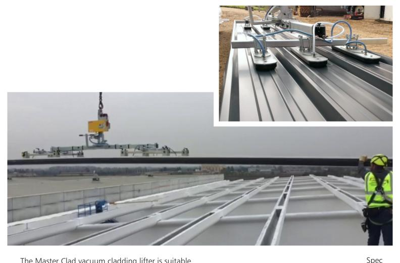
The Master Clad vacuum cladding lifter is suitable for the lifting and installation of a range of wall and roof cladding panels with varying length and shape. It can handle flat, micro rib or trapezoidal panels using adjustable vacuum pads to suit your requirements.
